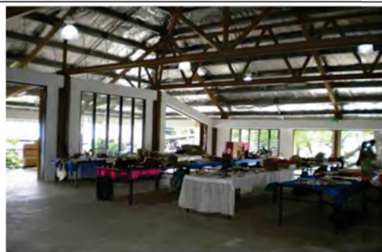
Image 53 Interior to be fitted with flexible partitions
