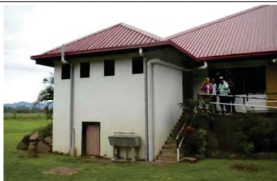
Image 54 One of two detached toilet-ablutions blocks
