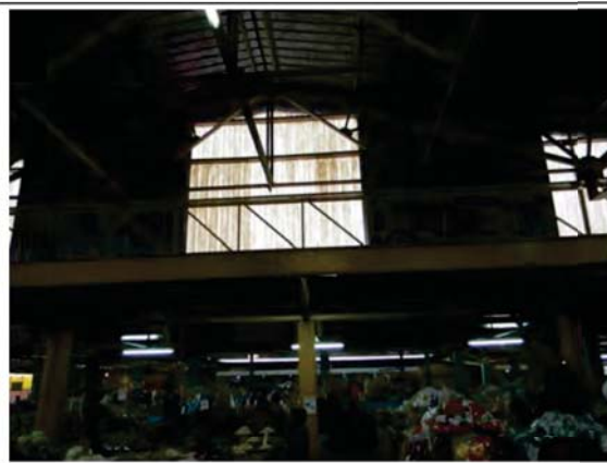
Image 3 Clerestory lighting main hall [D]
